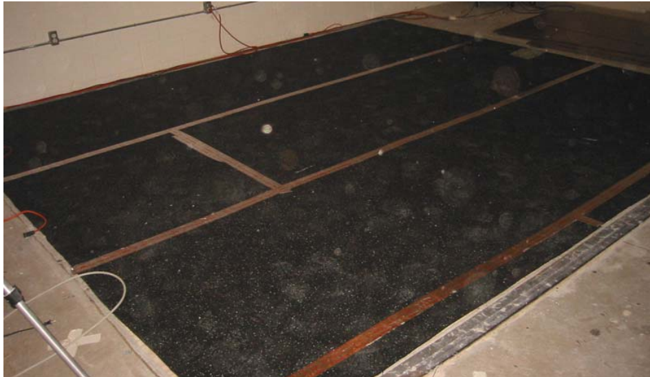
Figure 3: underlayment with foil tape
