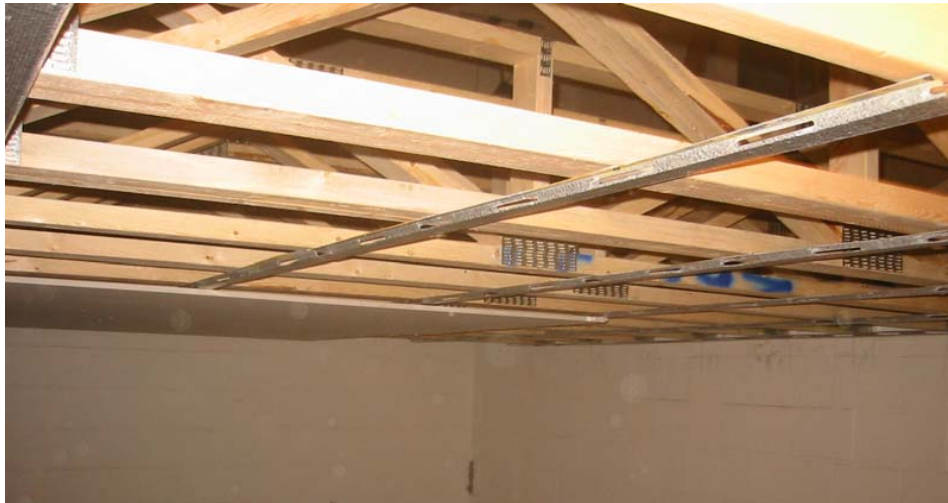
Figure 2: resilient channel and gypsum board ceiling
