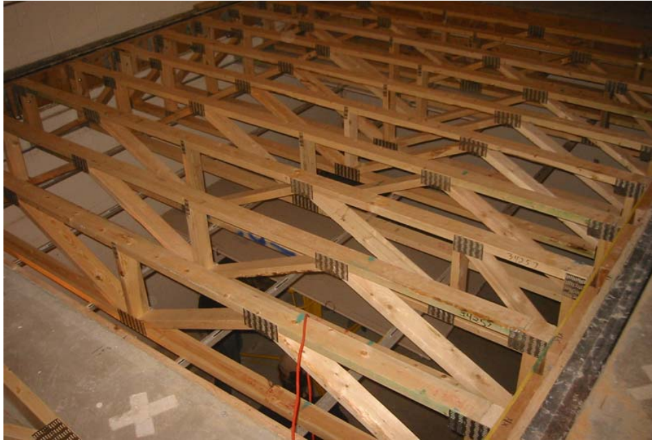
Figure 1: open-web truss joists
