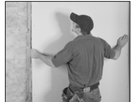
Figure 2.1: Install first layer of drywall
