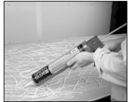
Figure 3.1: Apply Green Glue to the backside of second layer of drywall
