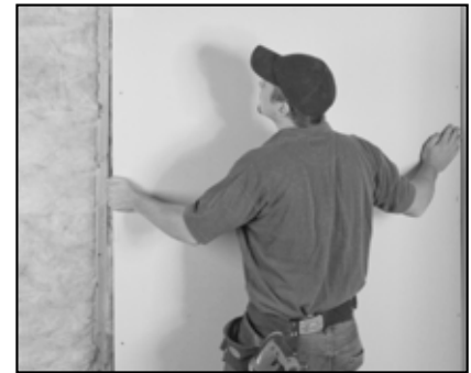
Figure 2.1: Install first layer of drywall
