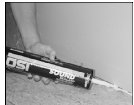
Figure 2.2: Use acoustical caulk along perimeter.
