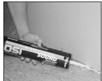
Figure 2.2: Use acoustical caulk along perimeter.
