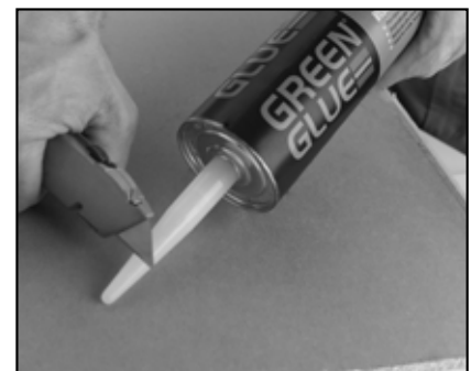
Figure 2.3: Cut a 3/8" opening in tube
