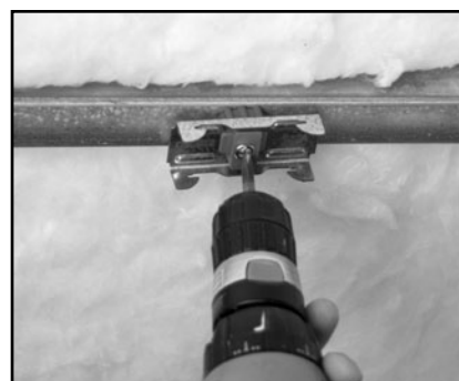
Figure 5.1: Screw A237R into joists
