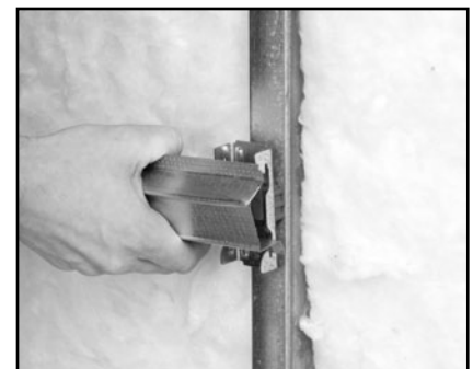
Figure 2.2: Snap hat channel into clip
