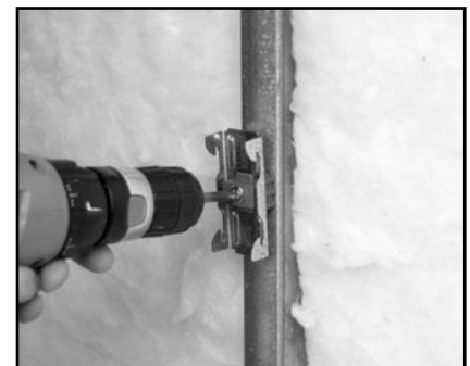
Figure 2.1: Screw clips into stud wall
