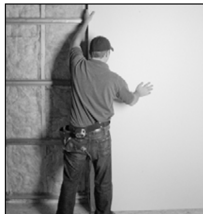
Figure 3.2: Install drywall vertically to hat channels
