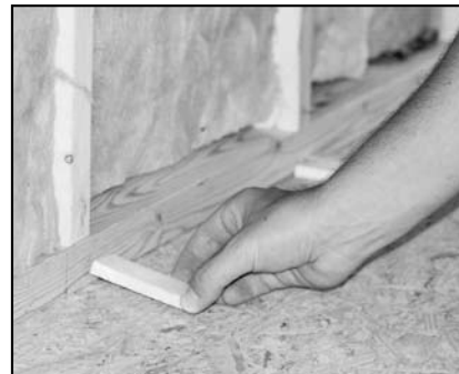
Figure 3.1: Place shims on floor in front of base plate
