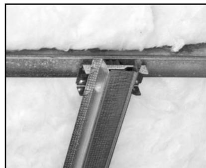
Figure 5.2: Snap Hat Channel into Clip
