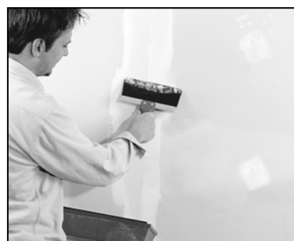
Figure 3.4: Tape and mud drywall
