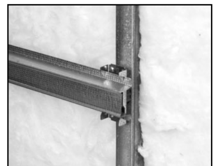
Figure 2.2: Snap hat channel into clip
