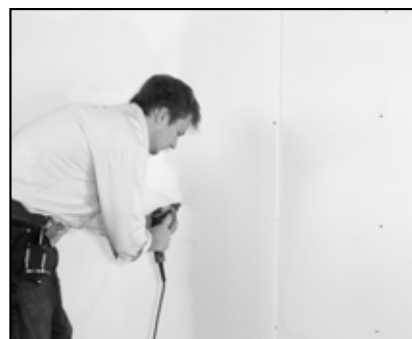
Figure 3.4: Secure second layer into place
