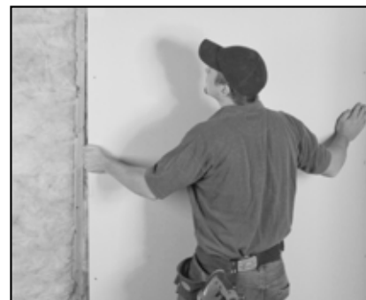
Figure 2.1: Install first layer of drywall
