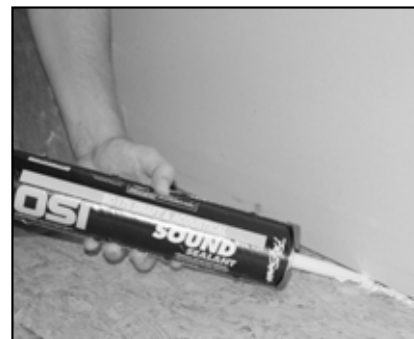
Figure 2.2: Use acoustical caulk along perimeter.
