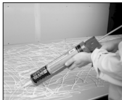
Figure 3.1: Apply Green Glue to the backside of second layer of drywall
