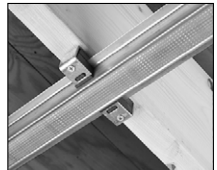
Figure 5.1: Screw SIC Clips into joist
