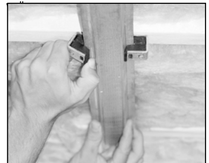
Figure 5.2: Snap Clip into hat channel
