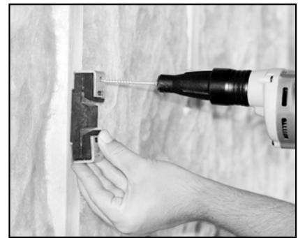
Figure 2.1: Screw SIC Clips into stud wall
