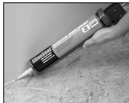
Figure 3.3: Use Acoustical Sealant around the perimeter and edges
