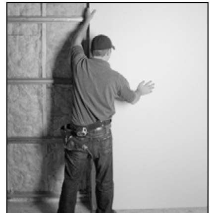
Figure 3.2: Install drywall vertically to hat channels
