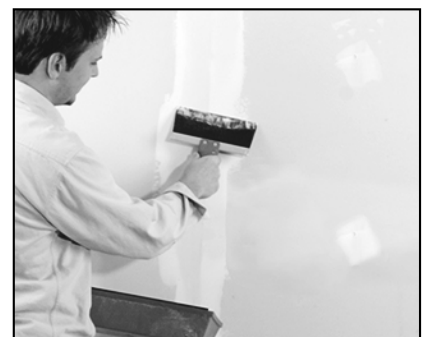
Figure 3.4: Tape and mud drywall
