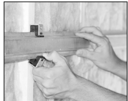
Figure 2.2: Snap Clip into hat channel
