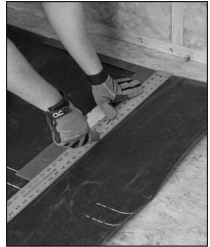
Cut Barrier to the appropriate length.
