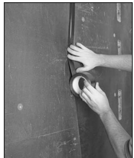
Tape vertical seams with foil or vinyl tape.
